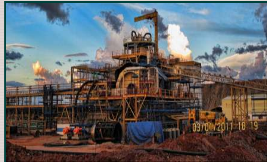
Mill & Cyclone Tower
