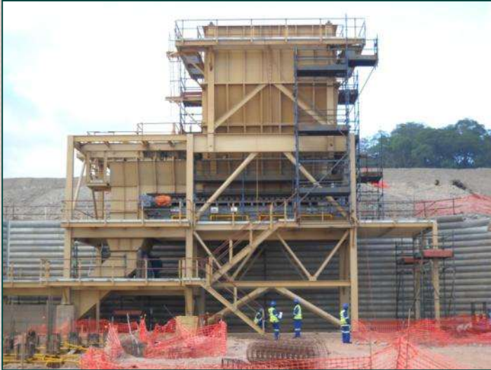
Crushing – MMD Sizer and ROM Pad
