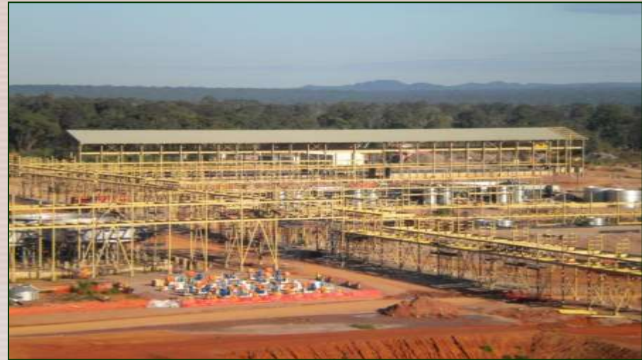
Electro-winning Tankhouse, SX and CCD thickeners
