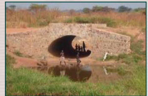
New Armco bridge - 2004
