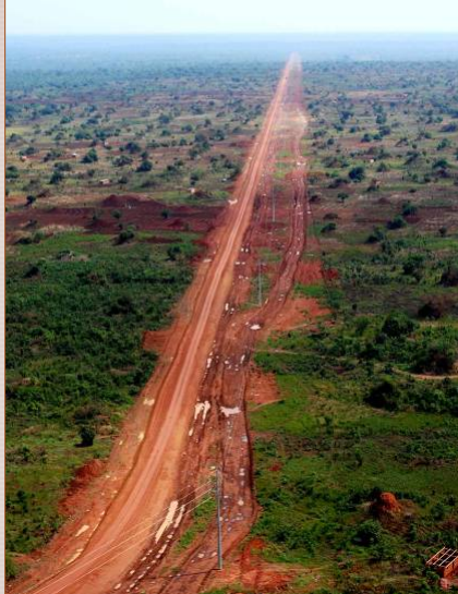
120kv Hydro-Electric Transmission Line Access Route
