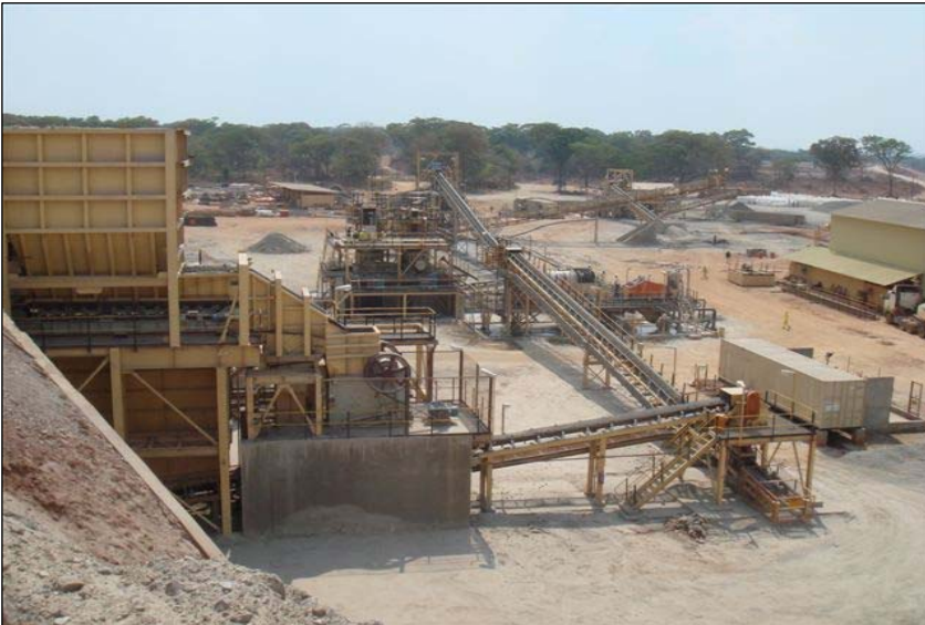
Kinsevere Mine Stage I Crushing and Screening Circuit
