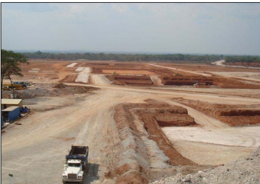
Clearing for Kinsevere Stage II Plant Showing Foundation Excavations
