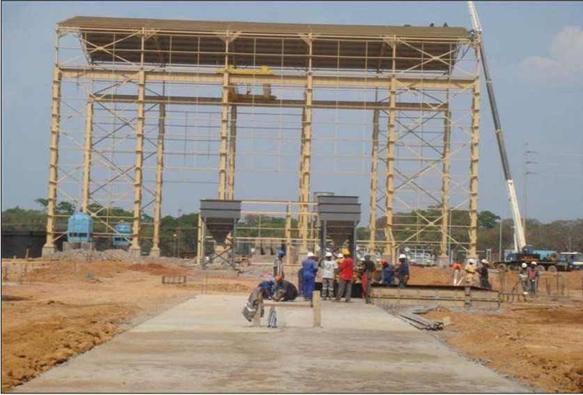
Kinsevere Stage I Electric Arc Furnace Building
