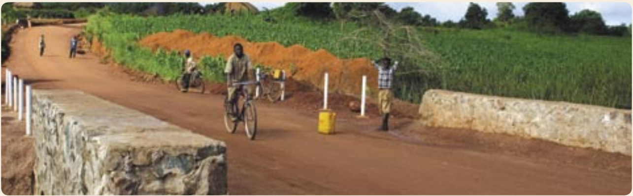
The new Kinsevere road & bridge
