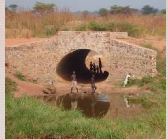
New Armco bridge
